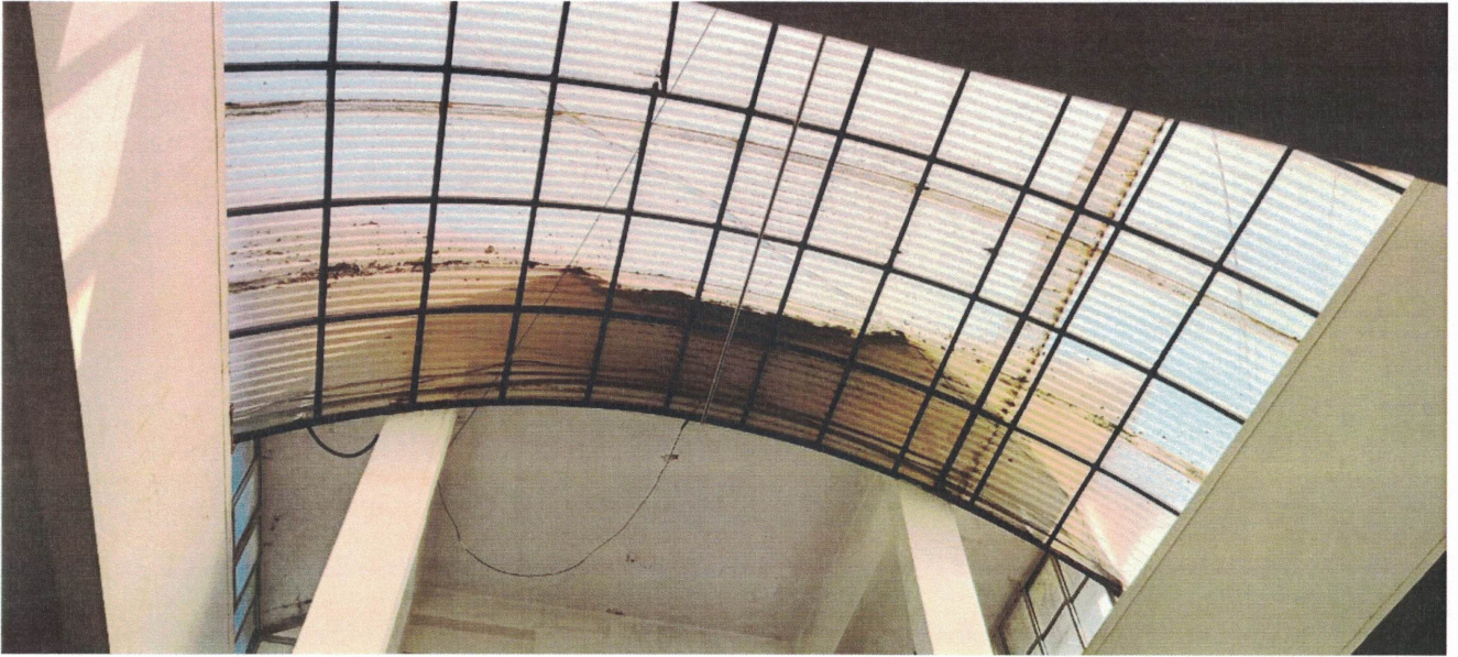
COVERED SHADE, IF REMOVED WILL HOTEL WILL BE OPEN TO SKY
